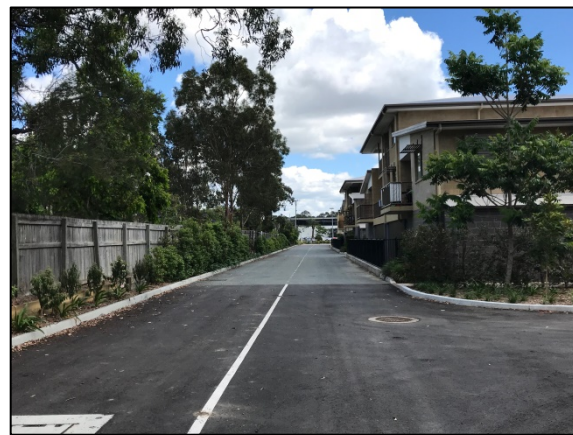
Internal road leading to Stage 4
